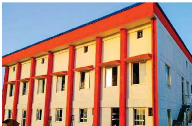
Mithirorhar Pump Station (VFD Building)
