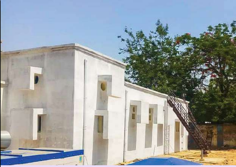
Control Building IOCL at Jhushi Prayagraj
